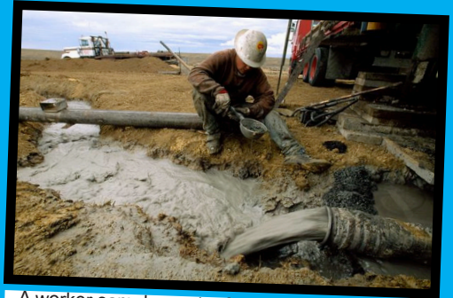
A worker samples water from a well at a coal bed methane drill site
